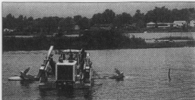
Machine digging trench under water.
